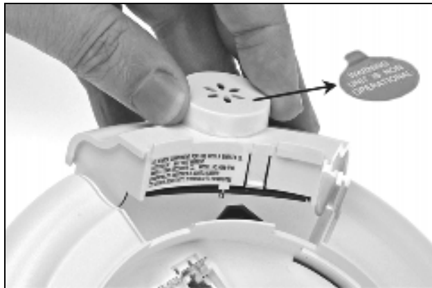
Figure 3-10. Installing the replacement CORC
