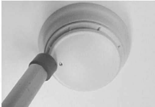
Figure 5-2. Magnet Test Location for 4098-9601, -9602, -9603, -9605 Smoke Detectors using 553-810 Magnet Tester
